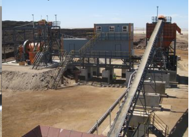
Main plant MCC & control room
